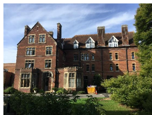
Homerton, Cavendish Building, red brick, Bath dressings, 1876- 1903
