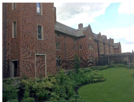
Wesley House, North Range (and Jesus West Court), red brick, Ancaster Striped Freestone dressings 1925-30
