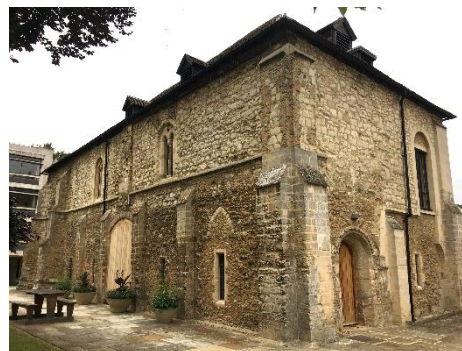
St John's, School of Pythagoras, Clunch and ragston rubble, Barnack and Clunch dressings, c1200
