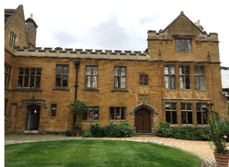
Trinity Hall Library Court, Master's Lodge, Ham Hill ashlar and dressings, 1852, 1890-2
